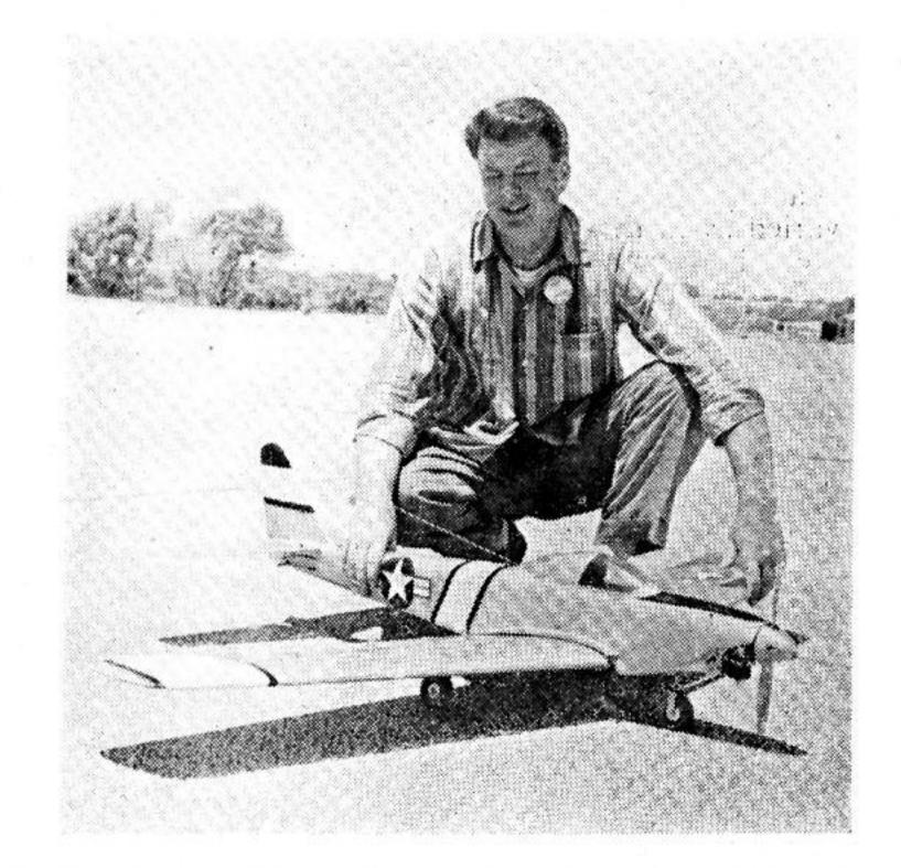
EIGHT-CHANNEL fully proportionate control, all simultaneous. Completely sealed in one unit to include servos and batteries (which can be charged "in situ").
